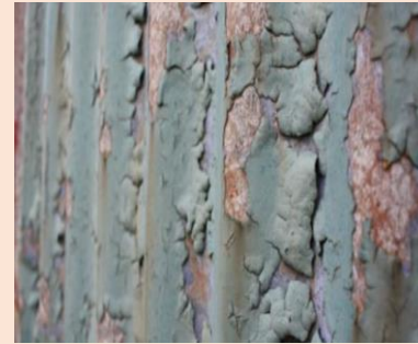
Multiple layers of paint
