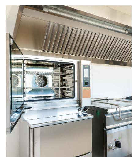
Pre–Engineered systems typically installed in the canopies above the cooking areas to prevent a fire entering the duct.
